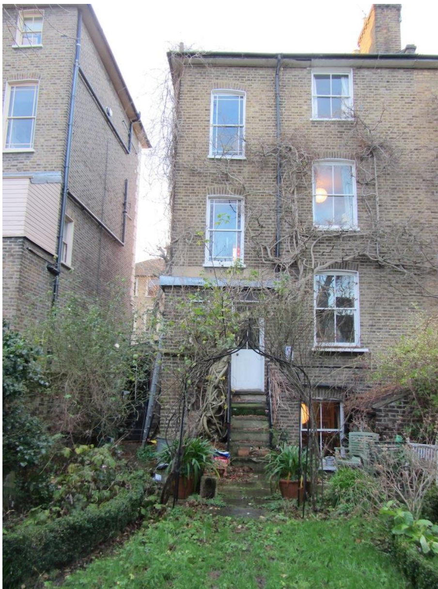
Photograph 3. Detailing the rear of the site
