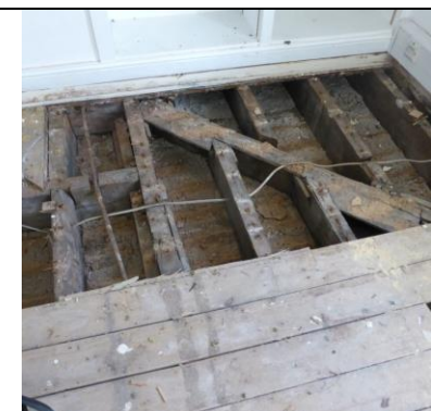
Fig 9 Floor structure in North East corner of The First Floor
