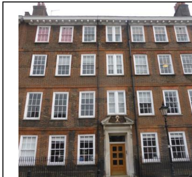
Fig 1 No12 Entrance & West Elevation to North/South Accommodation above
