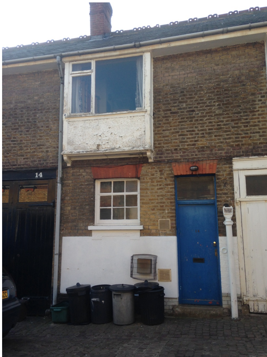
Figure 2: Existing Condition of Bay Windows at no. 14 Daleham Mews
