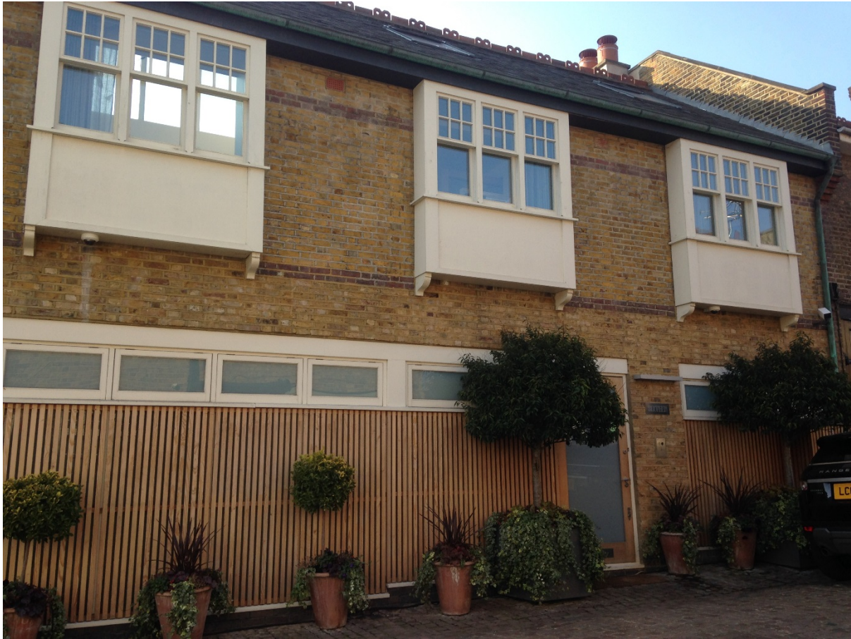
Figure 3: Sash Bay Windows at no. 16 Daleham Mews to be used replicated and used as a precedent.
