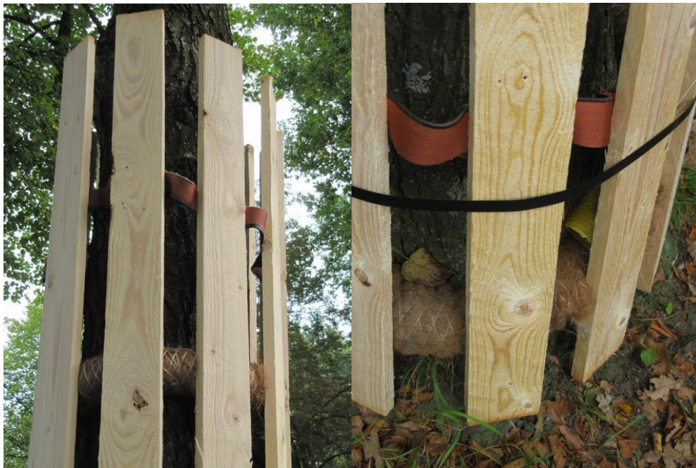
Figure 6 Insulated pipe inside planks, to protect trunks of T5 and T6.
