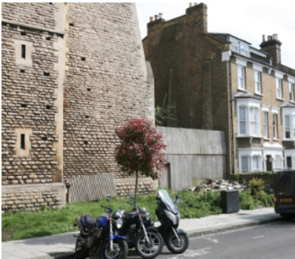
Existing situation with fence
