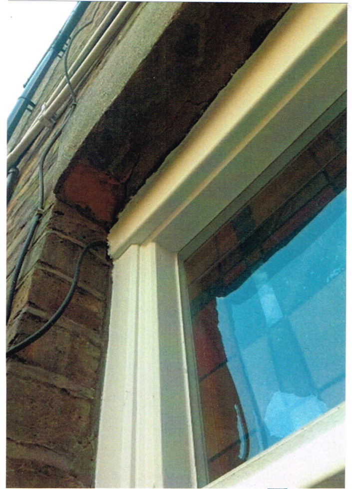
PHOTO 2 Render to Brick Arch Detail
