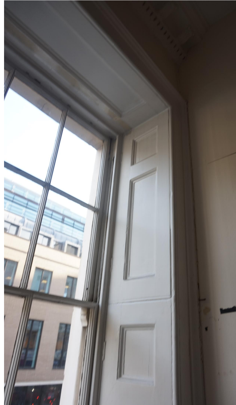
Ground, First and Second Floor - Showing panelling around windows
