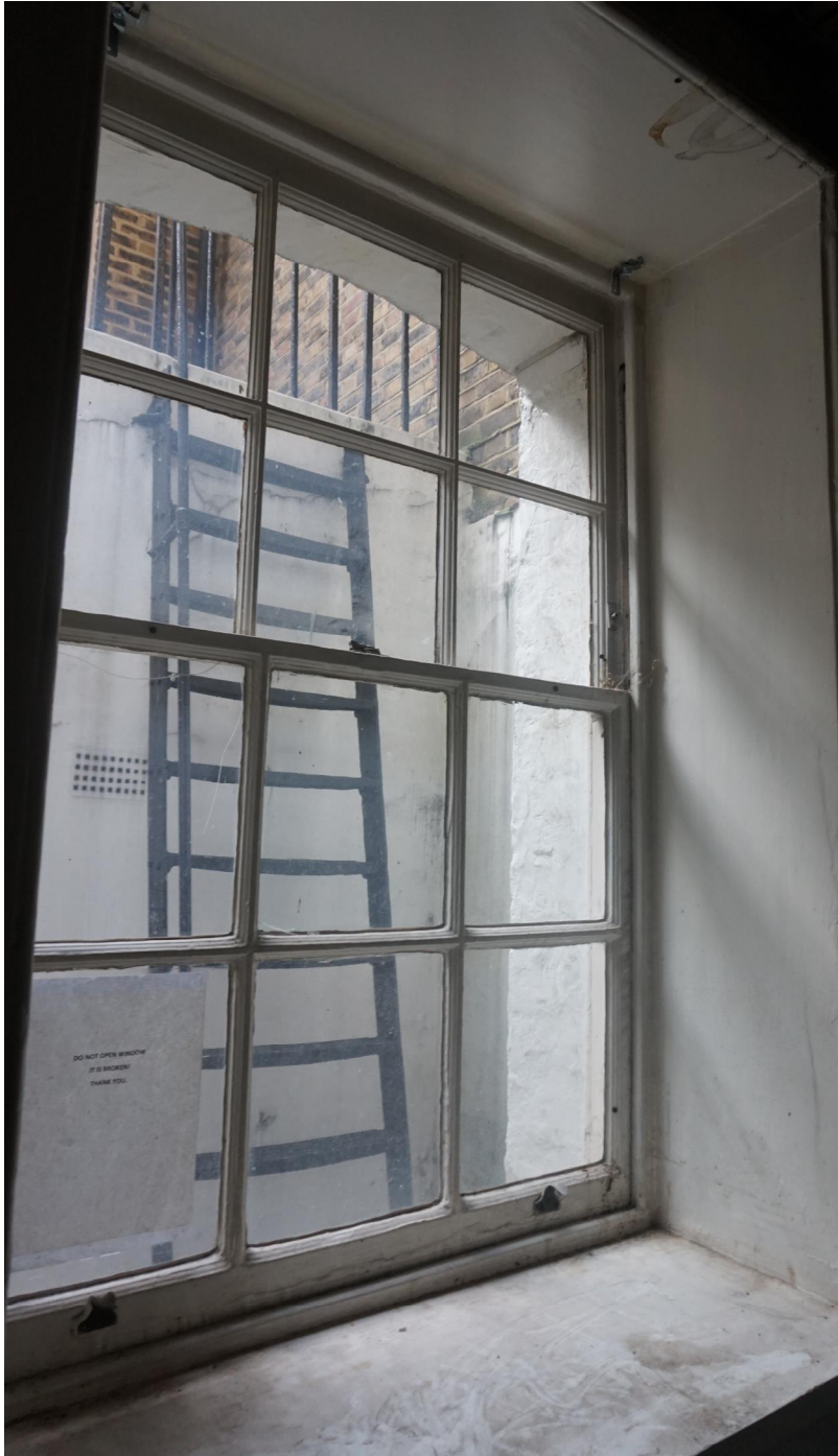
Basement Floor - Showing deep reveals
