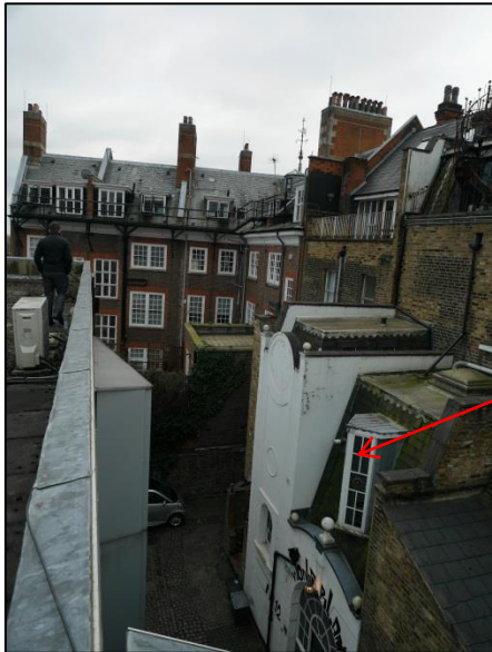
Figure 01 – Rear of 42-48 Rosslyn Hill
