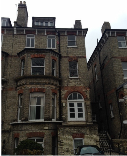
Image 1: Existing view of front elevation showing roof balcony
