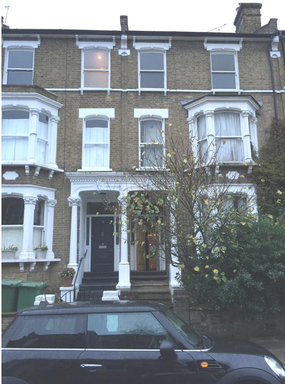
Photograph 1. View looking south east towards the site
