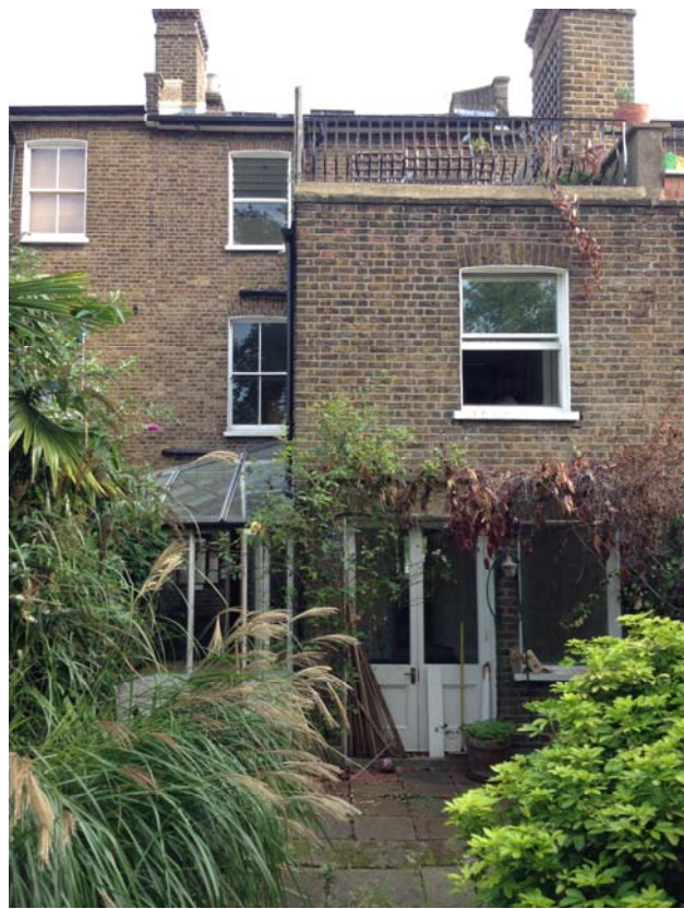
21 Boscastle Road - Existing rear elevation
