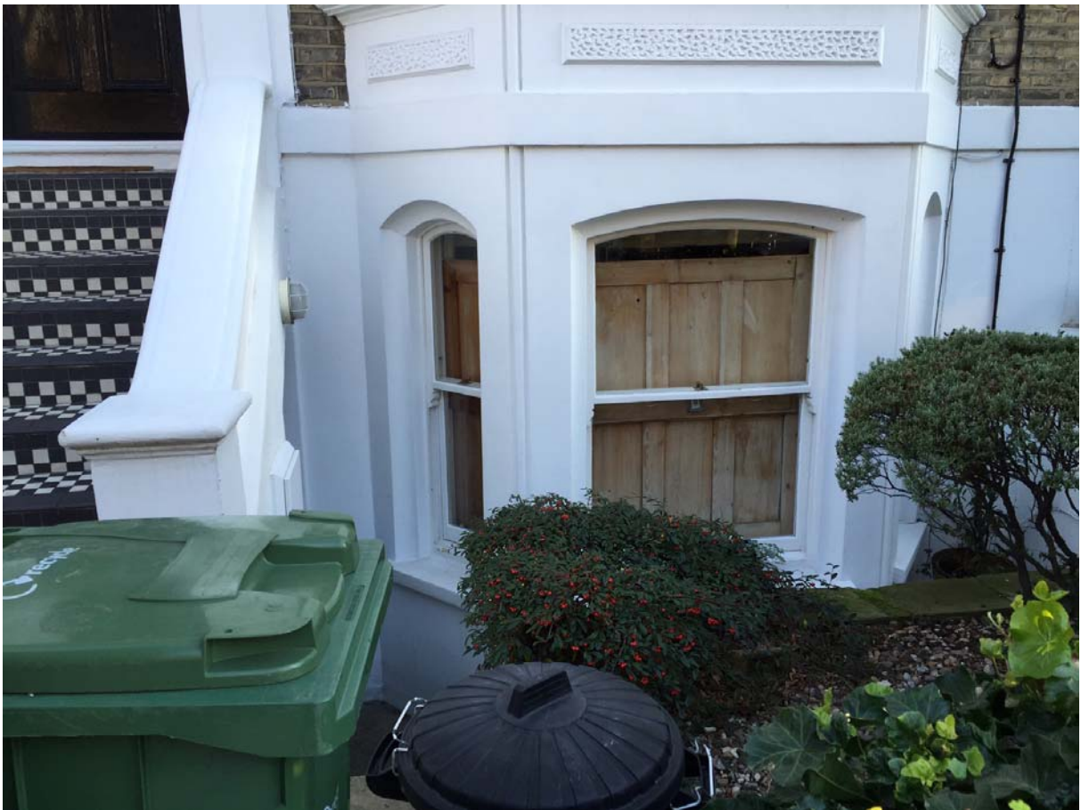
Basement level with bay window at 12 Boscastle Road.
