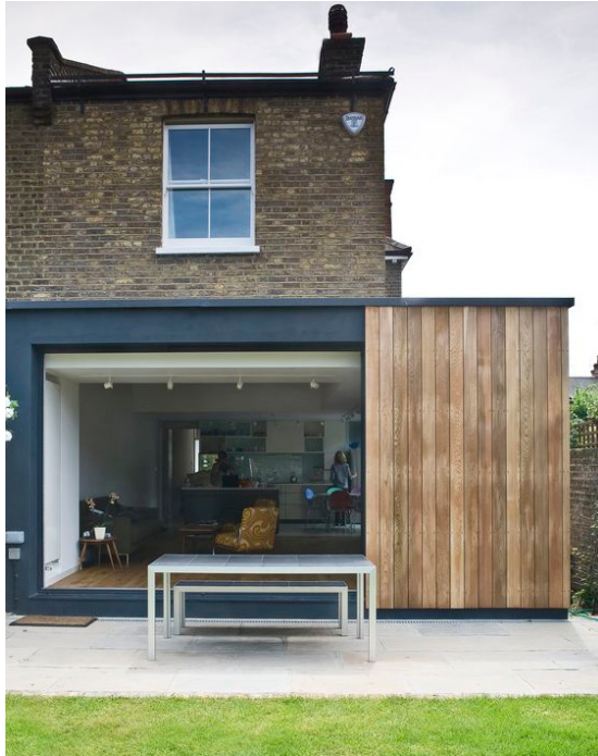
example of cedar cladding used with London stock brick.
