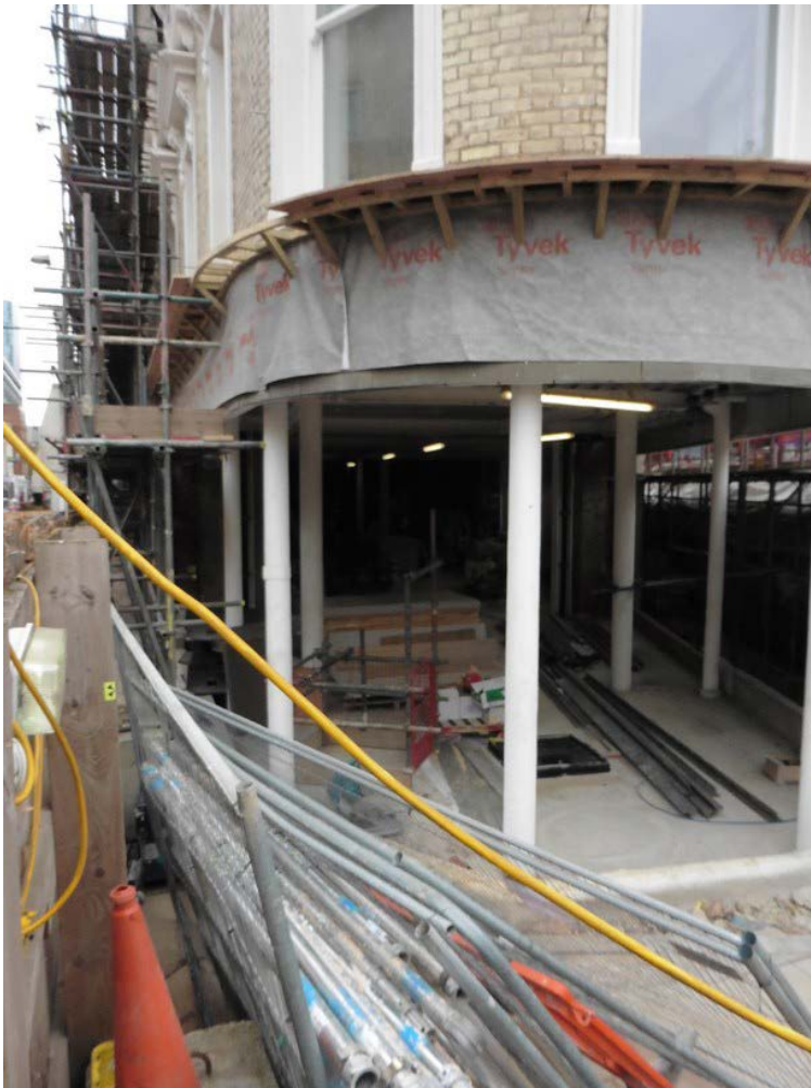
PHOTO 4: Shopfront Under Construction.
