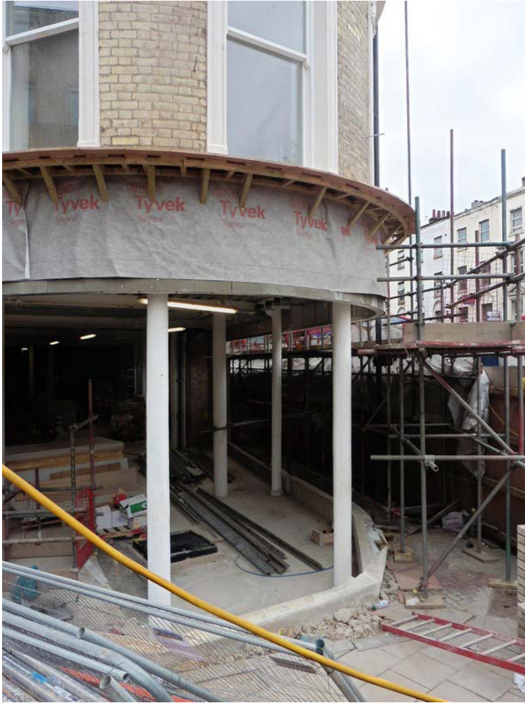
PHOTO 5: Shopfront under Construction.
