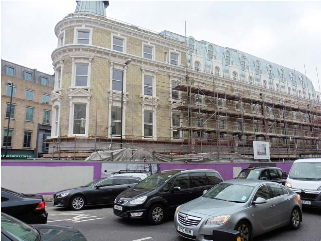
PHOTO 1: Grays Inn Road Elevation.
