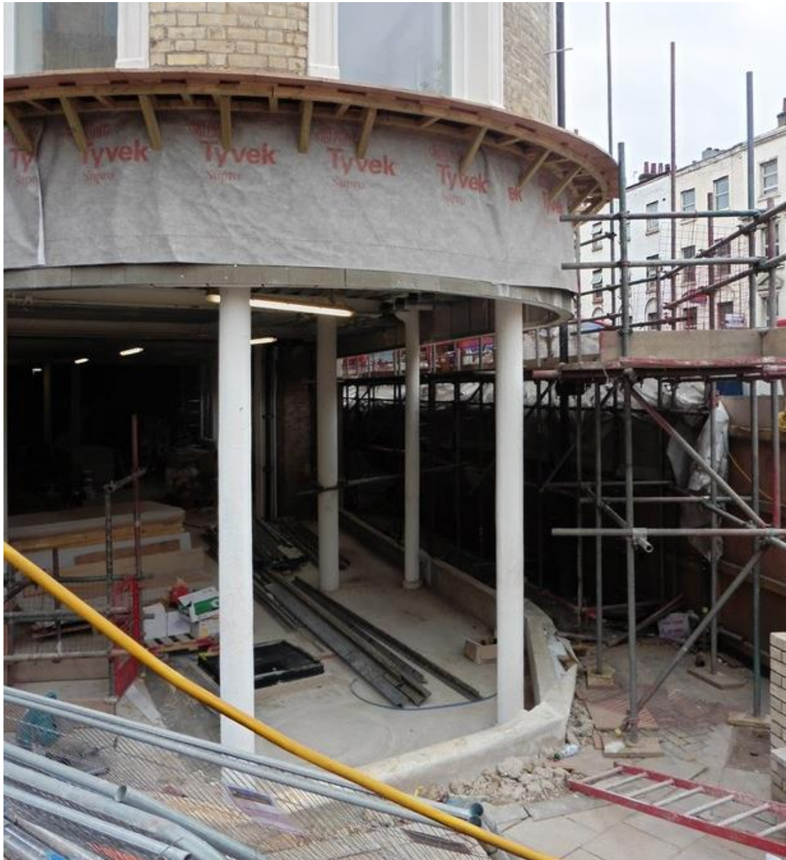
Shopfront Under Construction – August 2015
