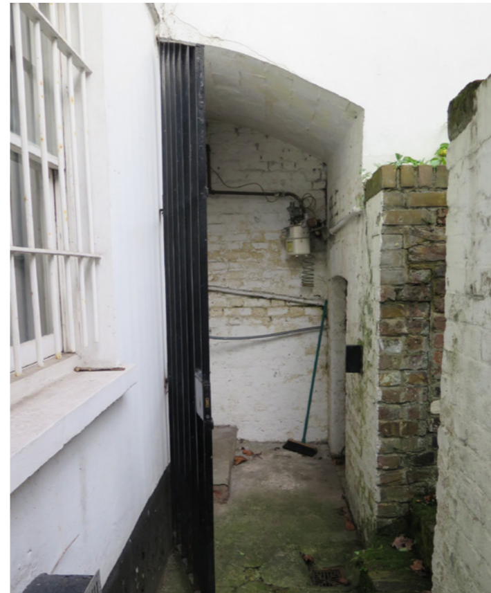
Lower ground floor entrance below steps (to be enclosed)
