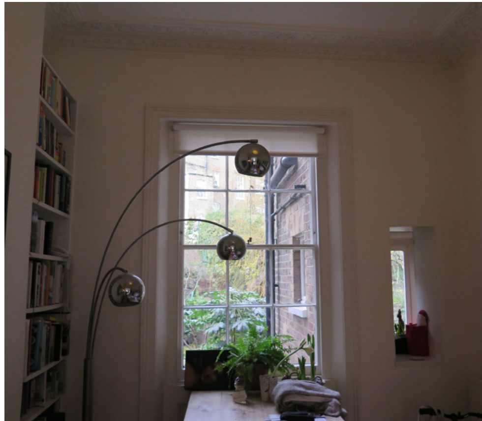
Rear window to kitchen (to be lowered - retaining architrave/surround) & adjacent hatch (to be infilled)
