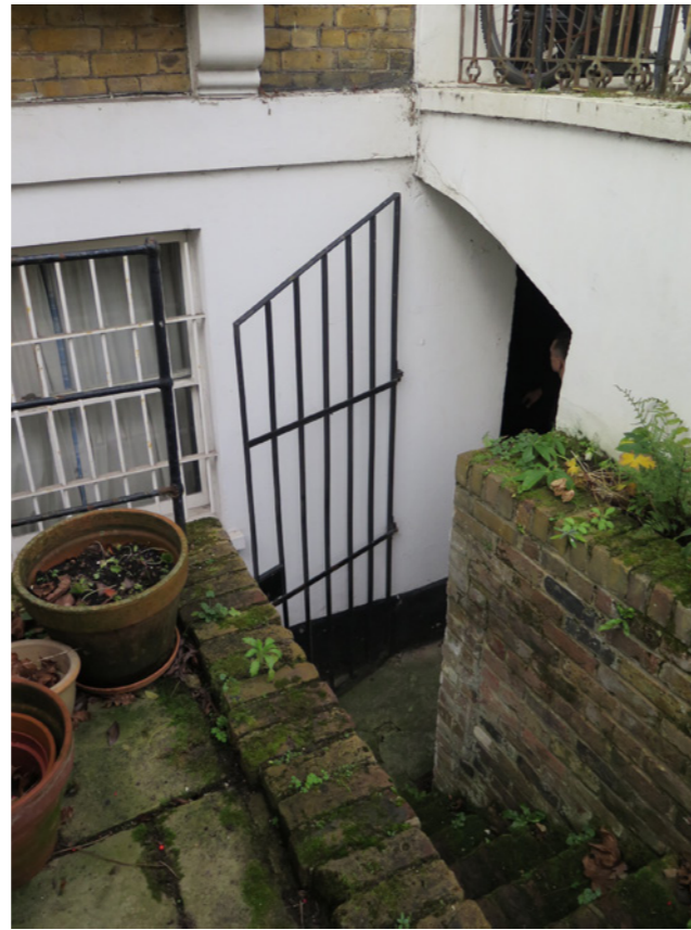
Lower ground floor entrance below steps (to be enclosed)
