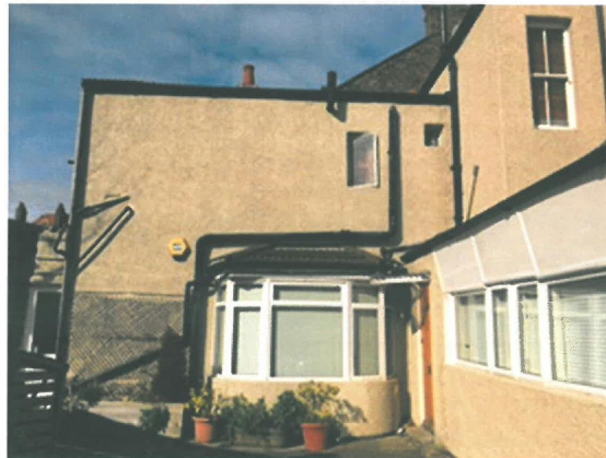
Entrance to the ground floor flat
