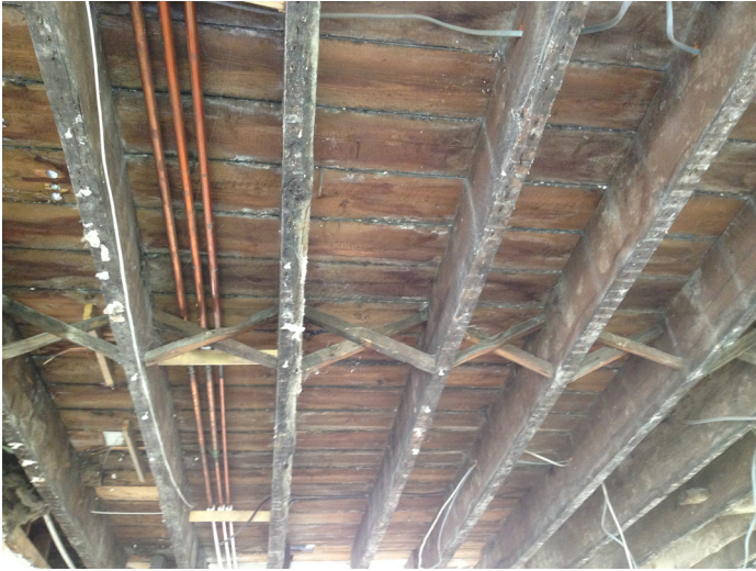
Two lines of herringbone strutting
