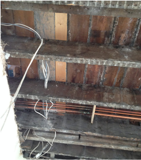
Two lines of herringbone strutting
