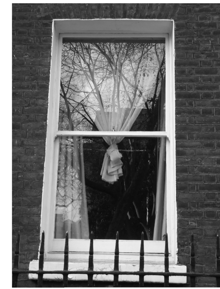
07 Existing Exterior W.0.2
