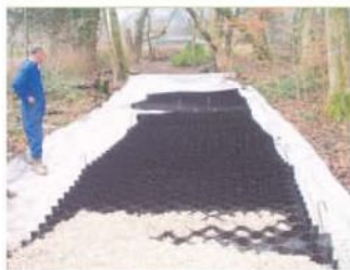
CellWeb during installation.
