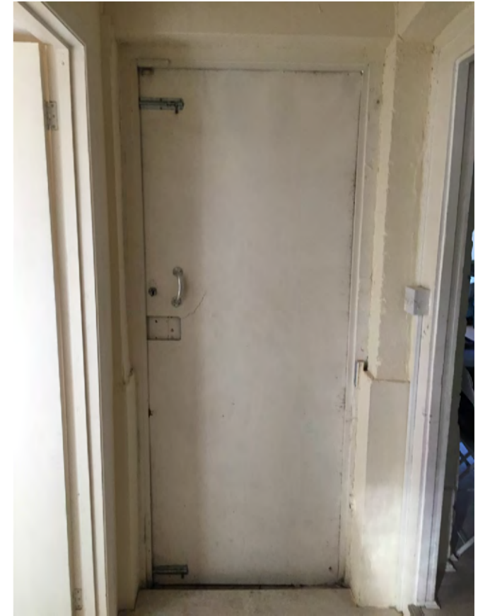
H) Existing door to Lower Ground Courtyard level to be retained.
