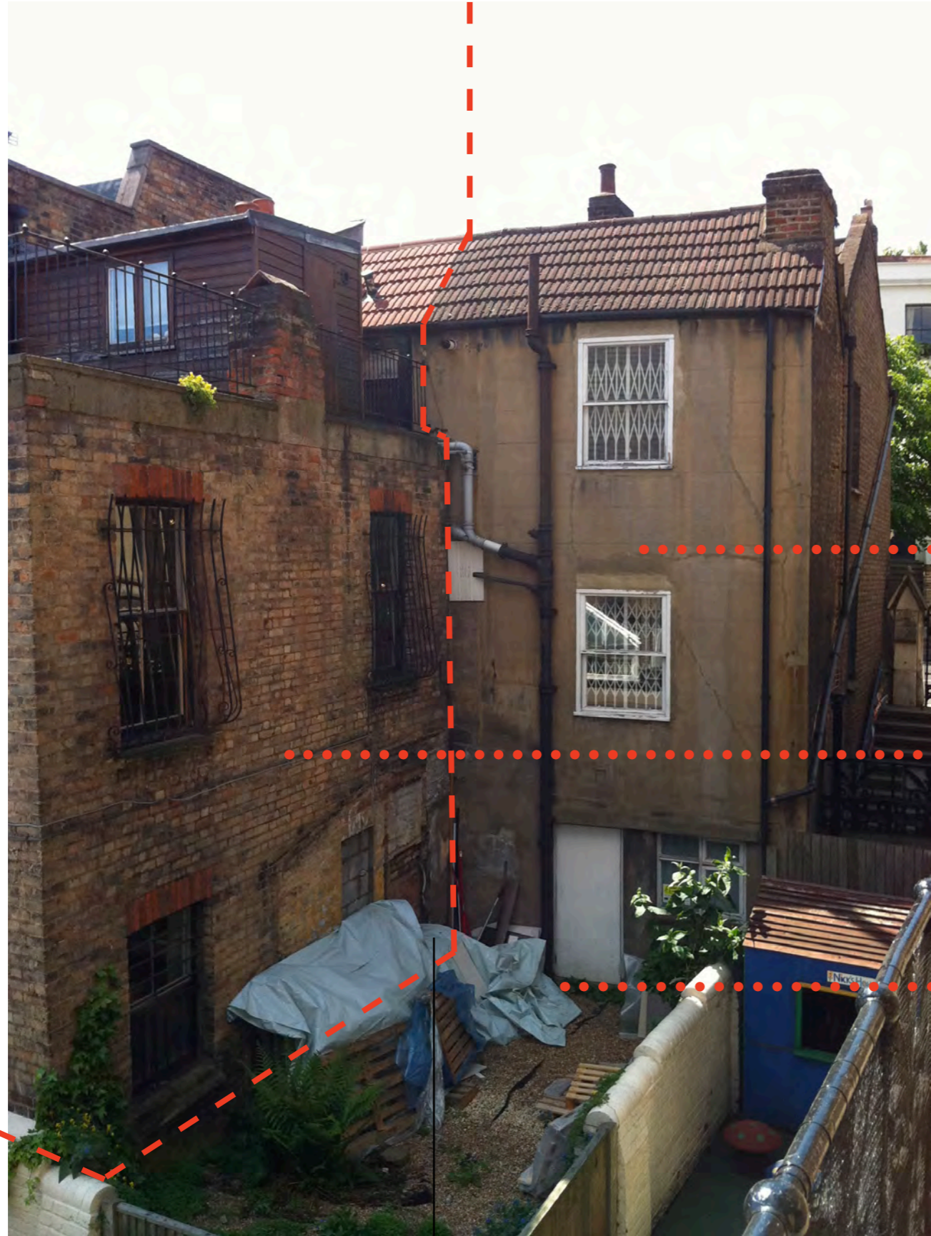
Rear of view of 82 Heath Street
