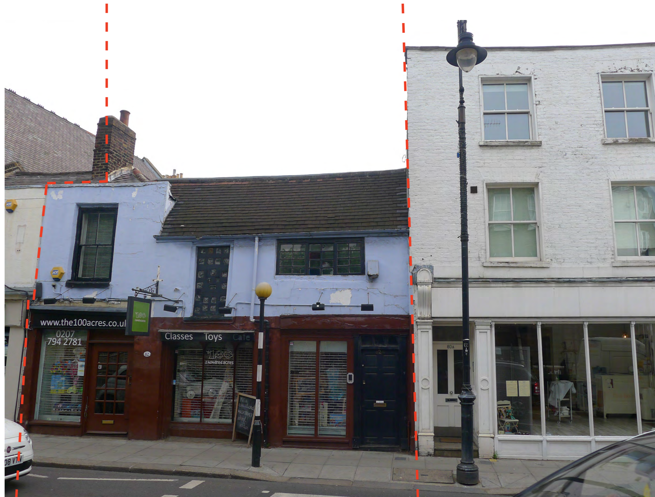
Front facade of 82 Heath Street, no change proposed to street elevation
