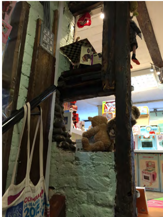
A) Original timber frames exposed to interior.
