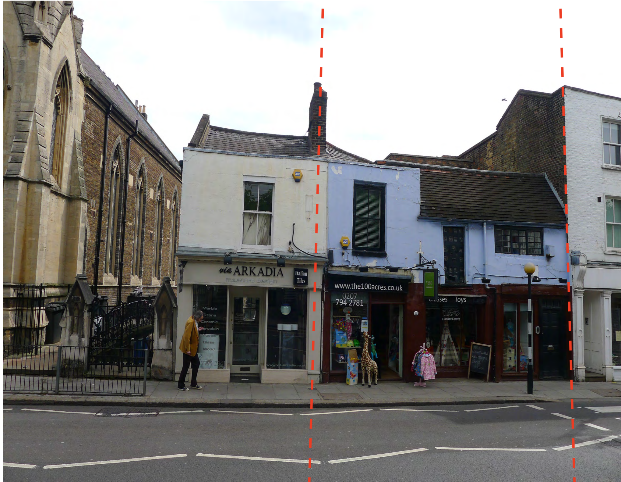
Front facade of 82 Heath Street, no change proposed to street elevation
