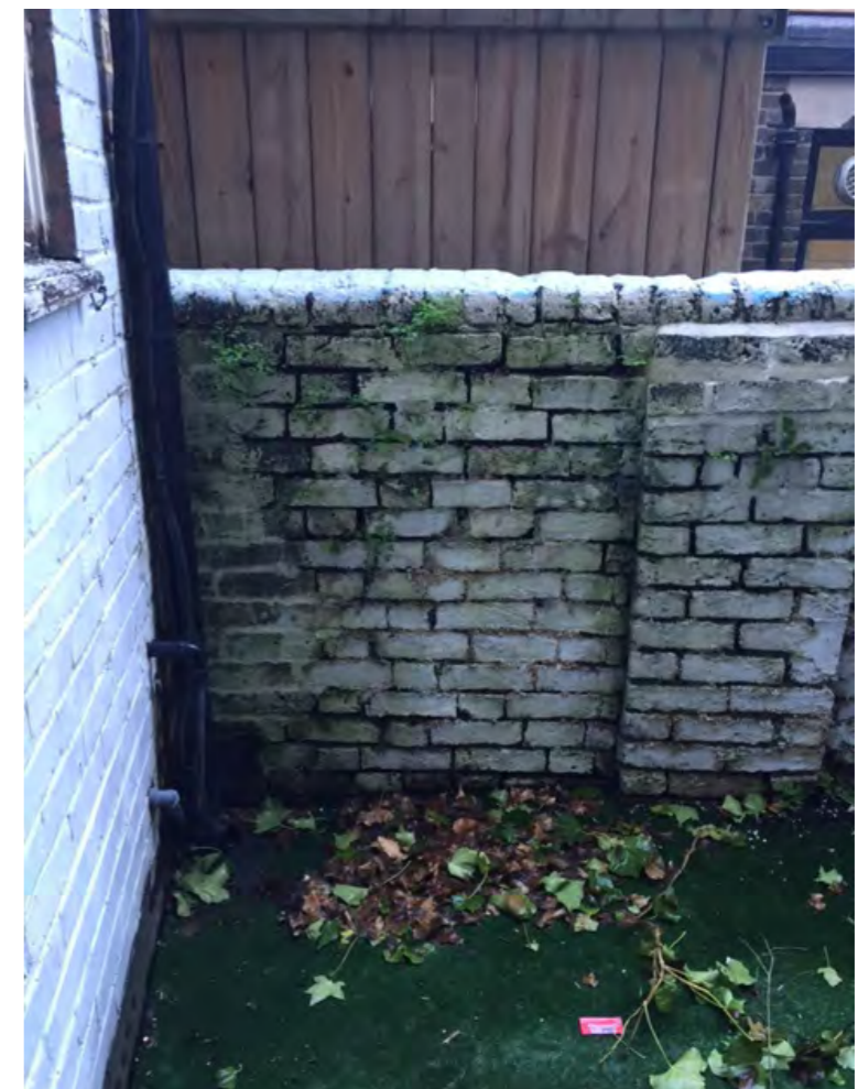
Low wall at back of site
