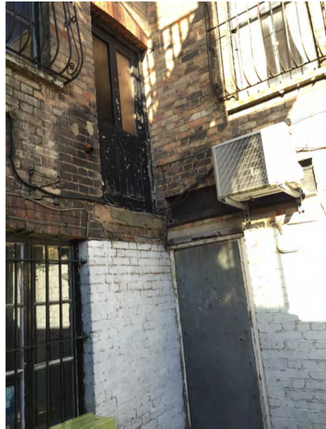
F) External view of existing door 001 to be reinstated on interior with addition of back painted metal staircase to exterior.
