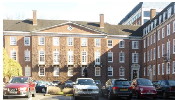
Fig 2 Existing parking Bays on the West side of South Square
