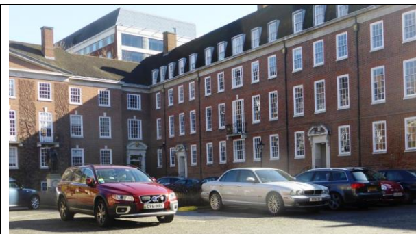
Fig 1 Existing parking Bays on the West side of South Square
