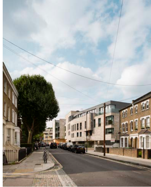
Fig.2 Existing view from Chester Road towards site
