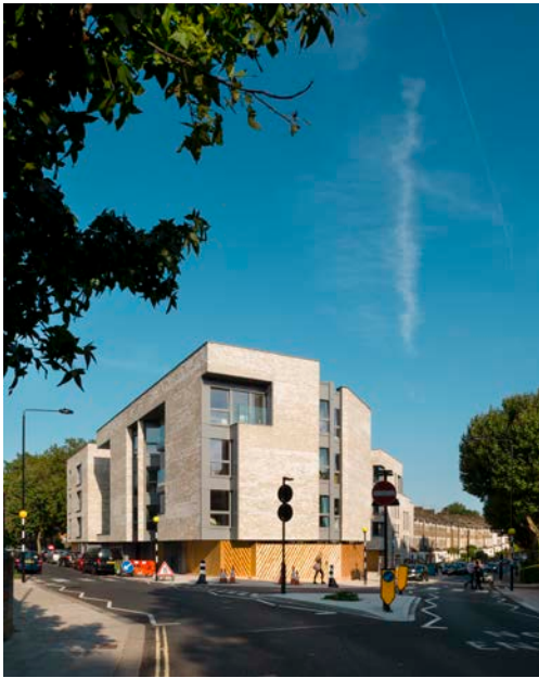
Fig 1. Existing view from Chester Road towards site
