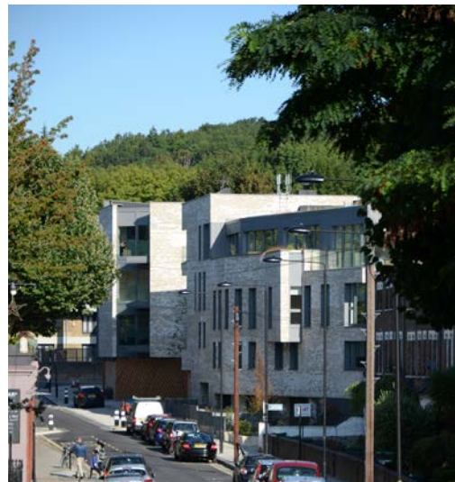
Fig.4 Existing view from Chester Road towards site
