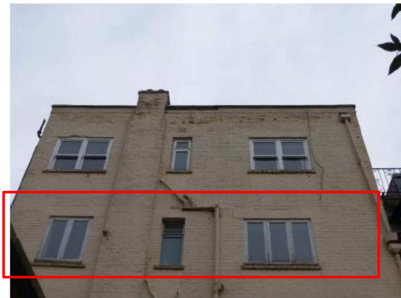
Photoplate 12 – Rear Elevation, second and third floors
