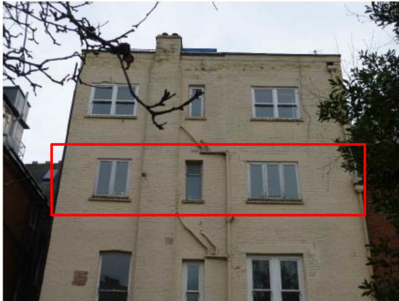
Photoplate 11 – Rear Elevation, first, second and third floors
