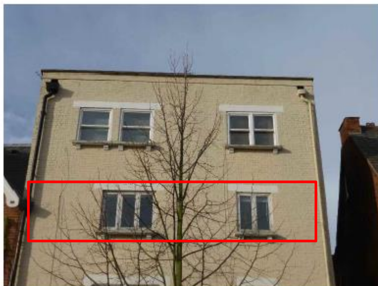
Photoplate 2 – Front Elevation, second and third floors
