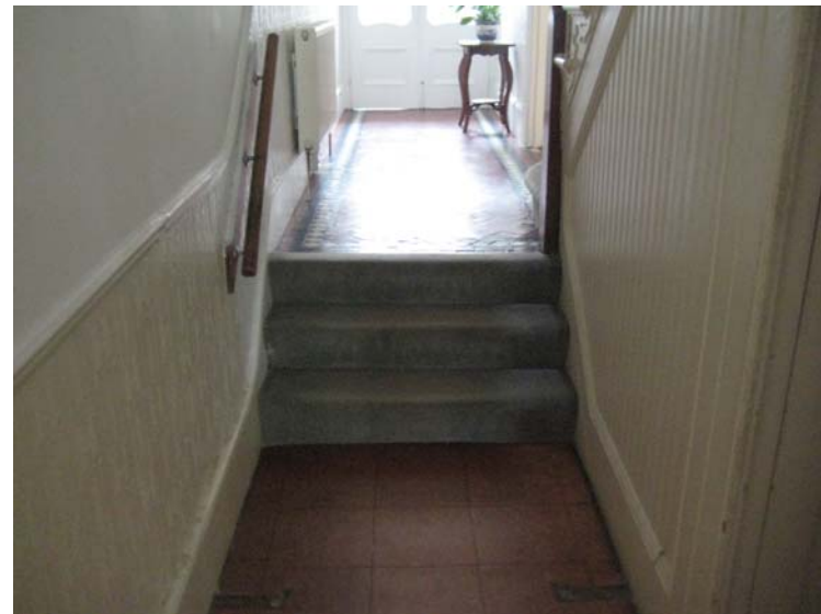
view of steps within common hall
