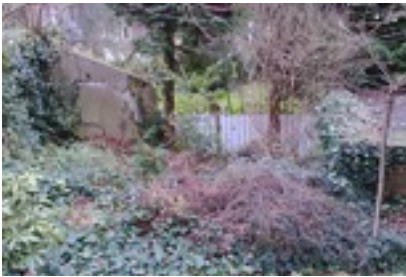
Fig 4. Southern boundary with old wall from previous building proposed to be demolished
