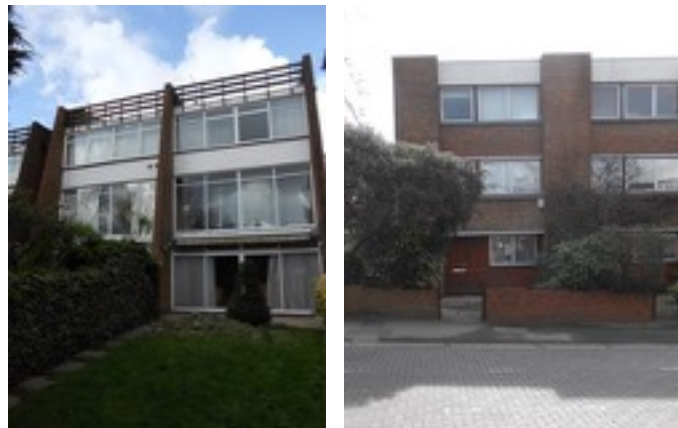
Fig 2. Rear and Front photos of the property
