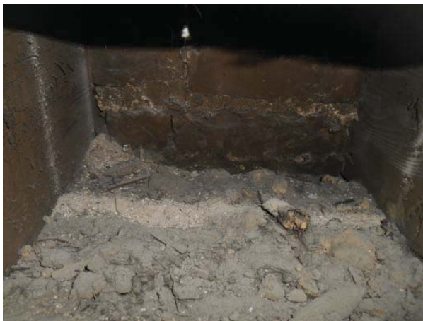
Photo 4: View of joists built into party wall.
