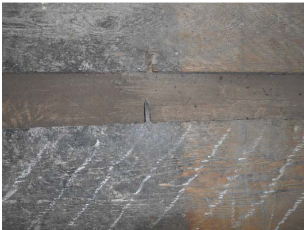
Photo 1: Timber pin recessed into top face of boards.
