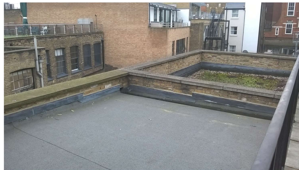
THIRD FLOOR'S REAR FLAT ROOF
