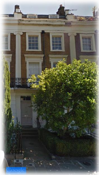
Fig 1: 42 Mornington Terrace – front facade
