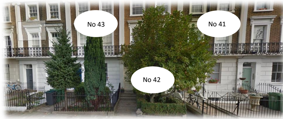
Fig 4: Frontage of No 42 Mornington Terrace and adjacent properties
