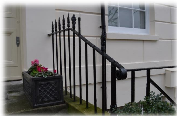
Fig 8: Railings flanking entrance steps
