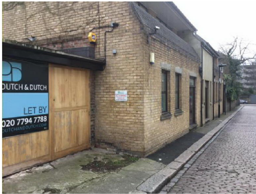
8. Camden Mews looking south with workshops and offices on left
