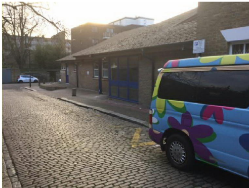
3. View of Camden Mews looking south with day hospital on right
