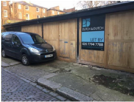
5. View looking north with two/three workshops on right
