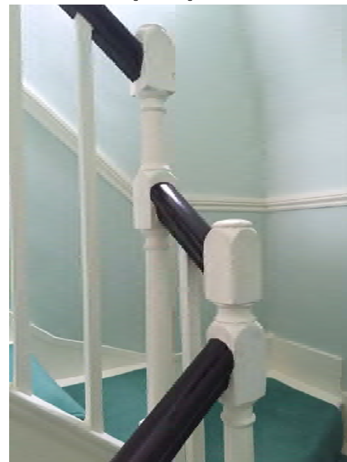
Plate 11: Original staircase newel posts second floor
