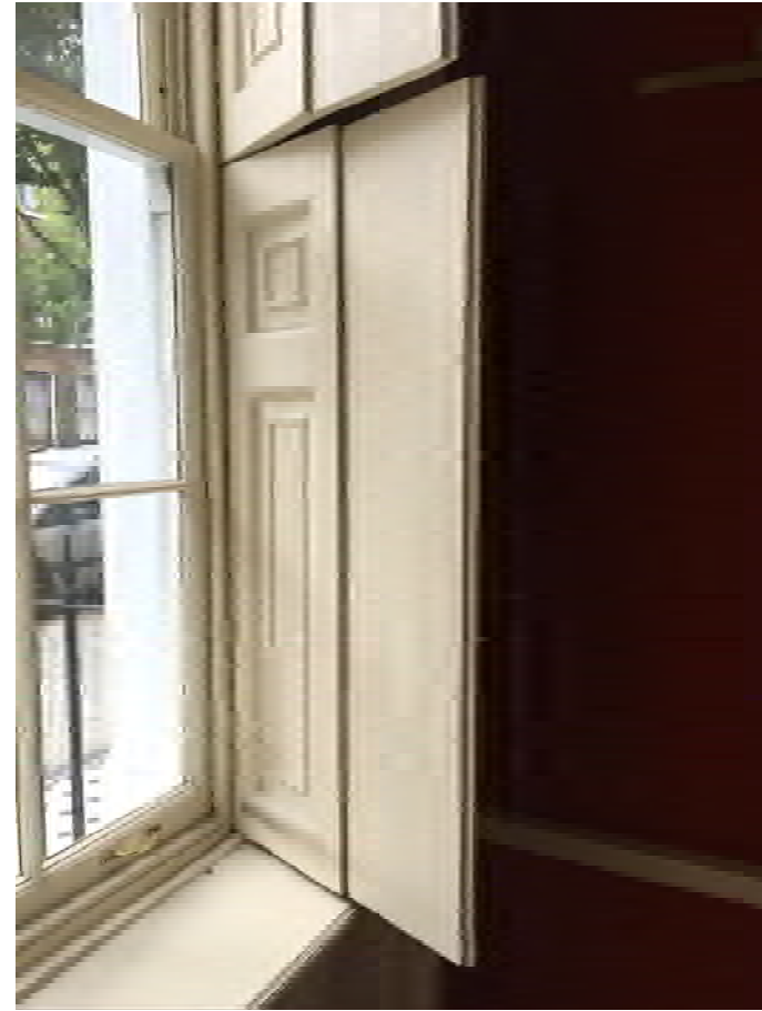
Plate 6: Front room ground floor original shutters
