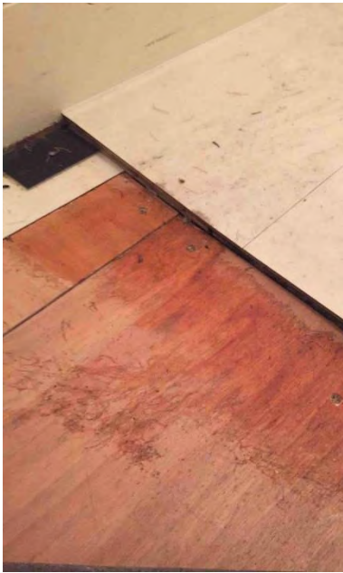
Existing vinyl flooring on plywood substrate in the entrance hallway.
