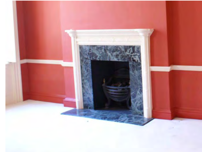
Existing fireplace to the front room to be replaced.
