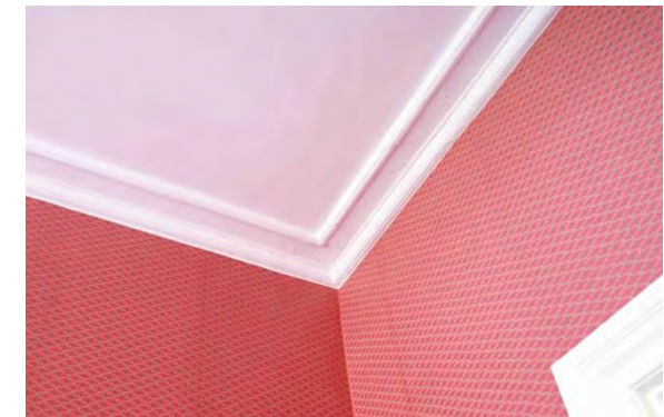
Existing cornice to the rear room to be retained.
