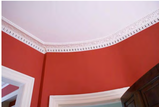
Existing cornice to the front room to be replaced.
