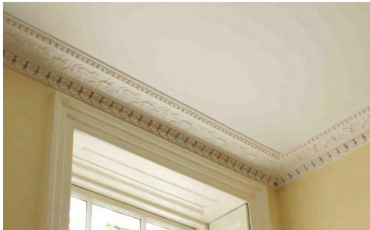
Existing cornice to the front room to be replaced.
