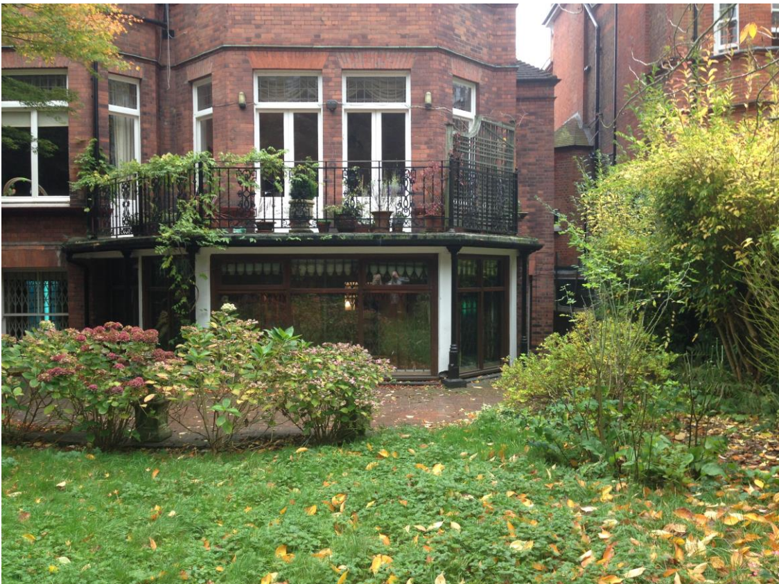
House Rear Façade with Garden
