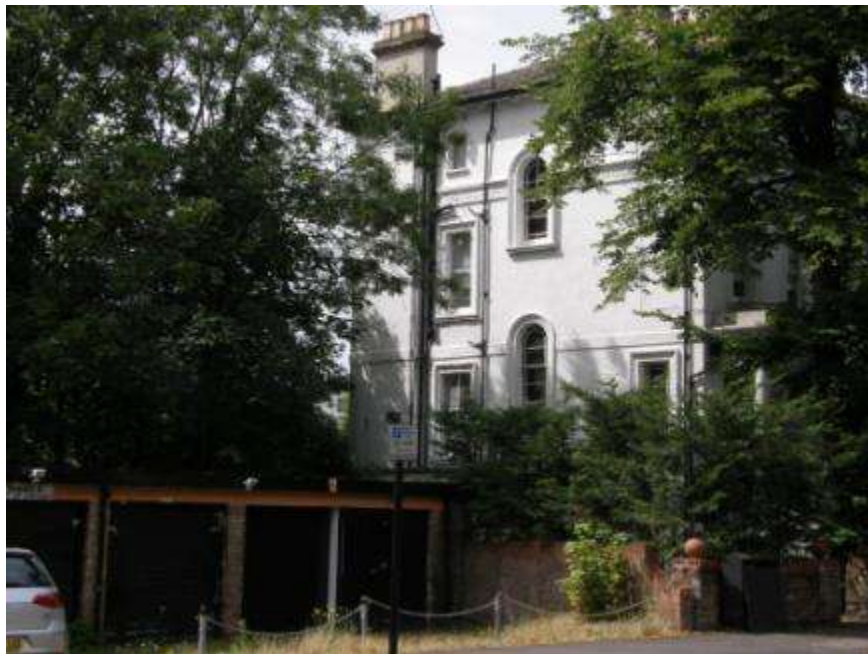
PHOTO 5. Mansion block on Abbey Road adjacent to the garages
