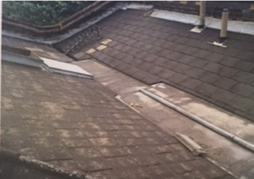
Image 2.0 Visual mock up showing proposed placement of sun pipe & ventilation kit
