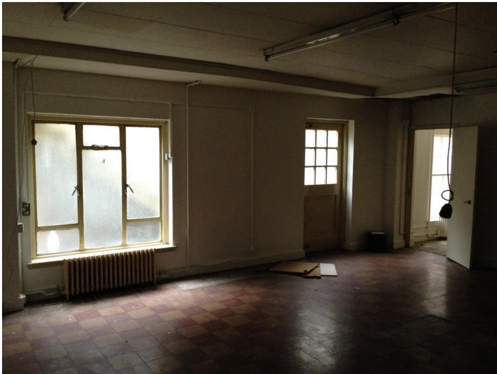
Examples of the interior of the basement
