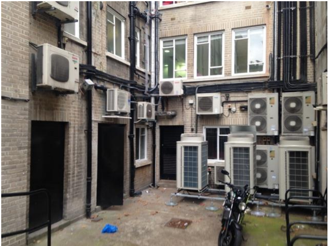
Existing Service Yard
