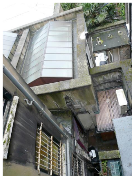
Existing lantern rooflights to 44 & 45
