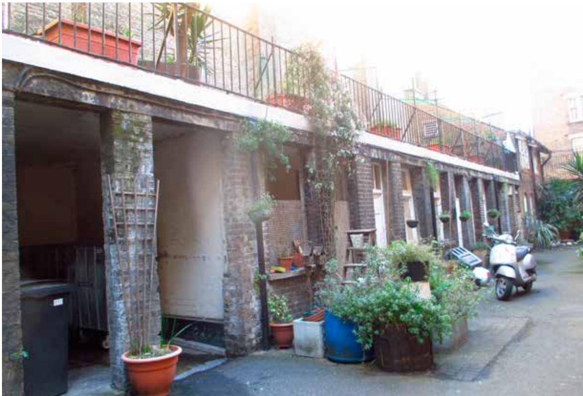
Fig. 3.6: View of the Aldwych Workshops elevation. It is proposed to salvage and reuse the iron railings, where possible.
