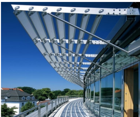
Figure 4. Solar PV Louvres on the South Facade
