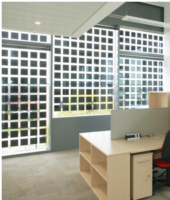
Figure 5. CPW Solar Glazing Installation, University of Warwick - Materials and Analytical Sciences Building
