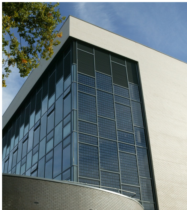
Figure 5. CPW Solar Glazing Installation, University of Warwick - Materials and Analytical Sciences Building
