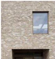
Buff multi brickwork
