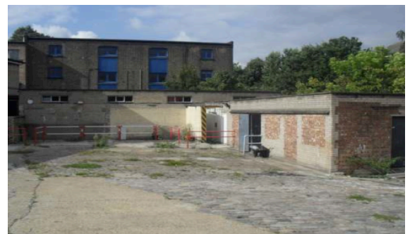
Figure 2.3: Existing buildings within the application site
