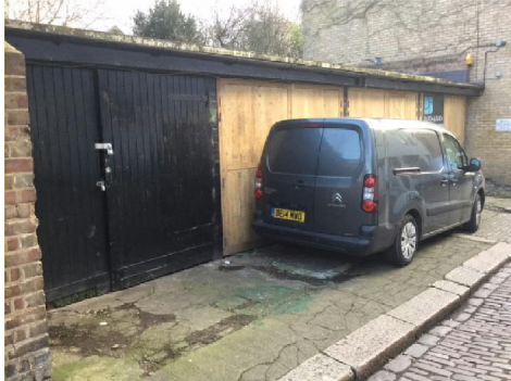
4. View looking south down Camden Mews with two/three workshops on the left
