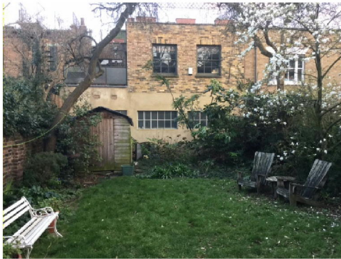
9. Rear view of 9 Camden Mews from the garden of 160 Camden Road
