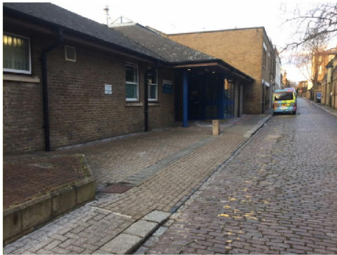
2. View of Camden Mews looking north with day hospital on left
