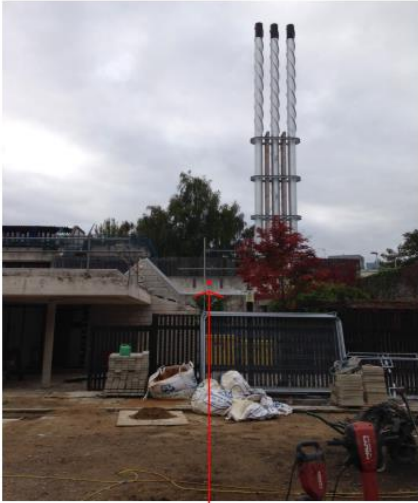
LOCATION OF CHP FLUE EXTRACT 220mm diameter, 150mm projection from wall
