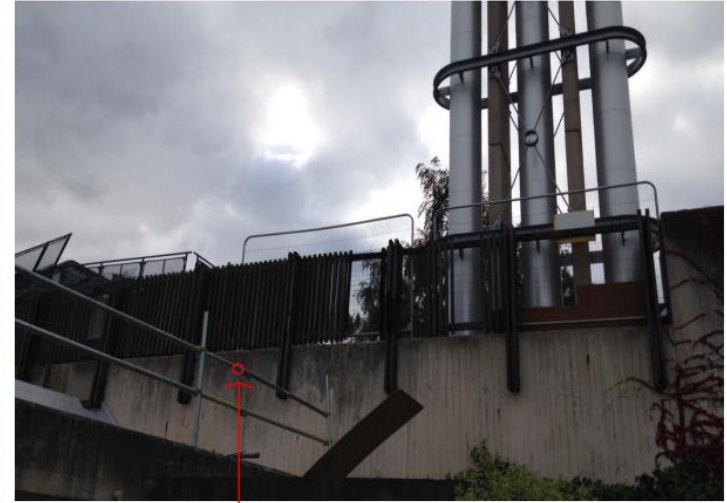
LOCATION OF CHP FLUE EXTRACT 220mm diameter, 150mm projection from wall
