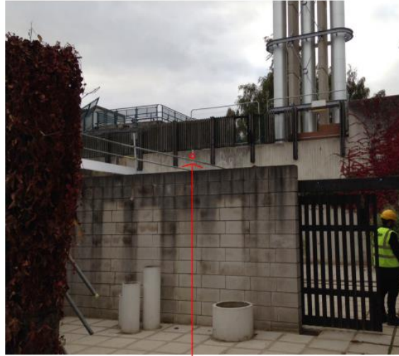
LOCATION OF CHP FLUE EXTRACT 220mm diameter, 150mm projection from wall
