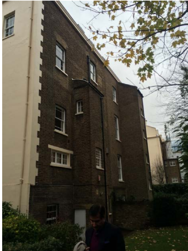
Existing rear facade
