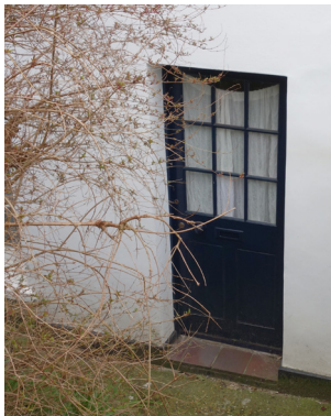
1. Existing main door to basement flat
