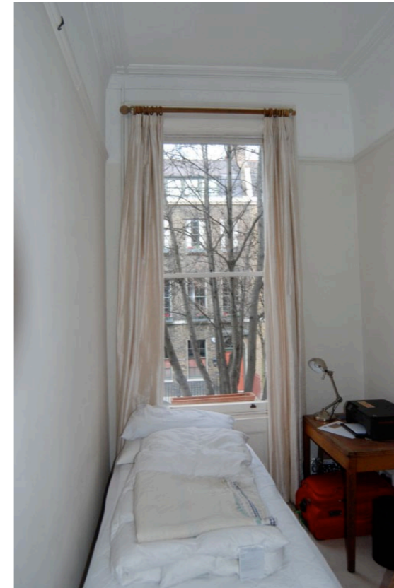
Partitioning (to right) forming study bedroom to be removed to re-open three-bay reception space
