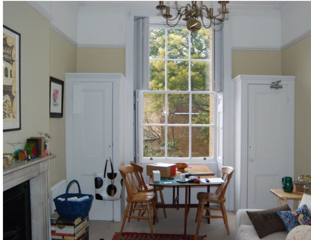
Fire compartment door structure (to right), to be removed and replaced by a fire protected corridor providing means of escape from the rear bedroom. 'Matching' cupboard (to left), to be removed
