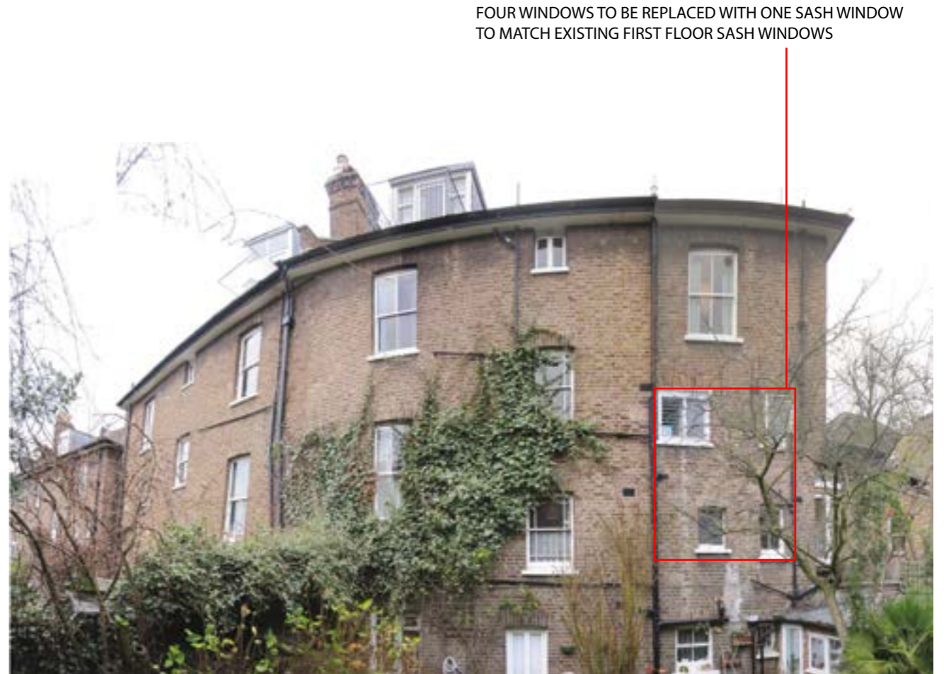
Fig 3.D Rear Elevation of number 22 South Hill Park Gardens and adjacent properties
