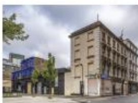
Existing view from Museum Street
