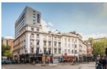
Existing – corner of New Oxford Street & Museum Street
