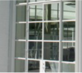
W10 Metal casement window PPC finish, histoglass double glazing; Crittall or similar
