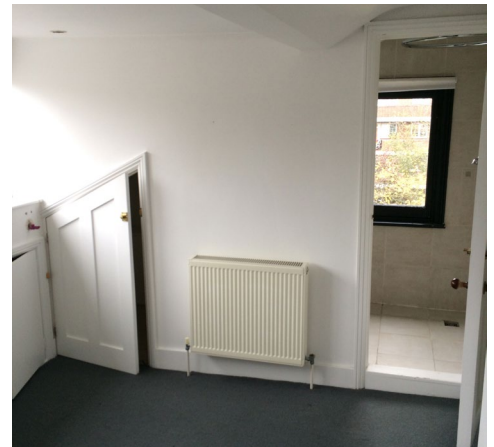
Second floor square edge skirtings.
