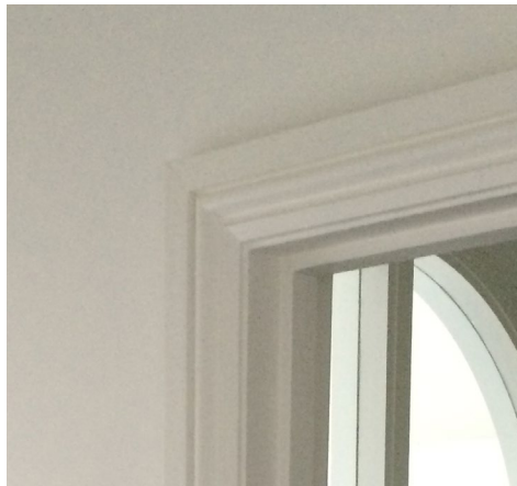
First floor architrave.
