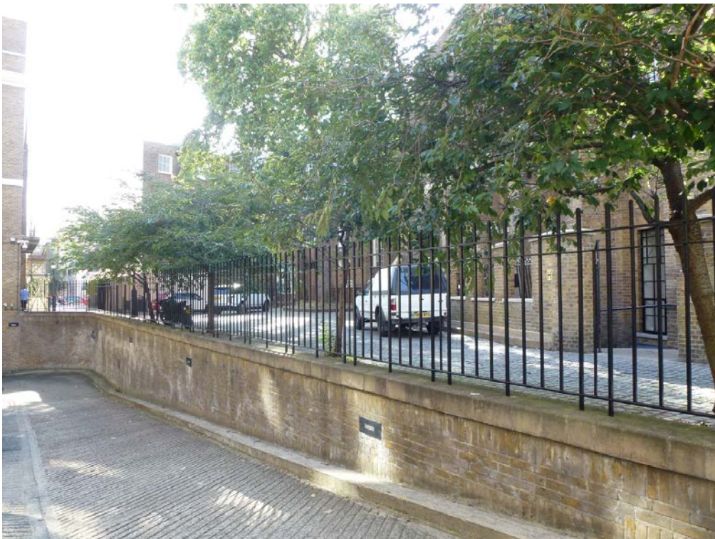
Image 12 Image of T1 – T4 looking South West with Basement carpark ramp retaining wall in foreground.
