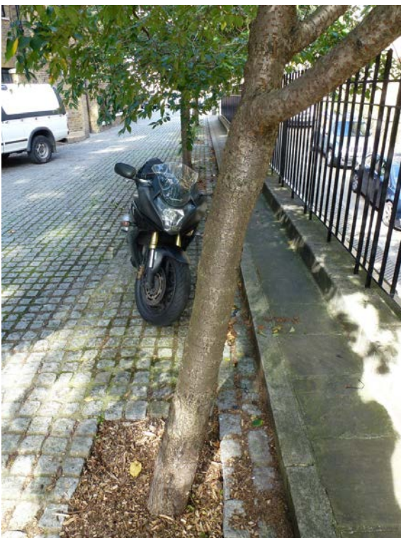
Image 02 Image showing T1 trunk leaning East.
